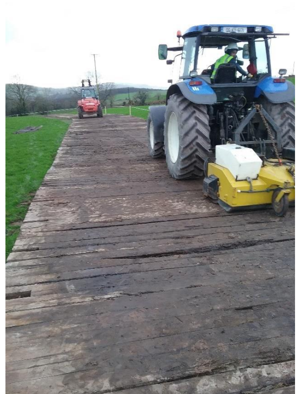
Figure 5 - Temporary timber roadway (Bog matt)
