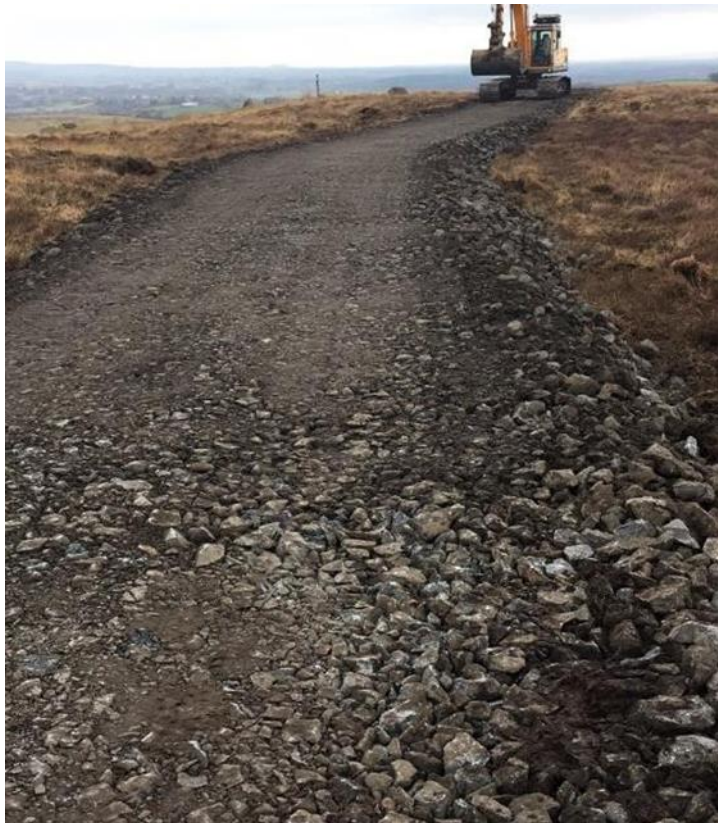
Figure 10 - Typical Windfarm Access Road.
