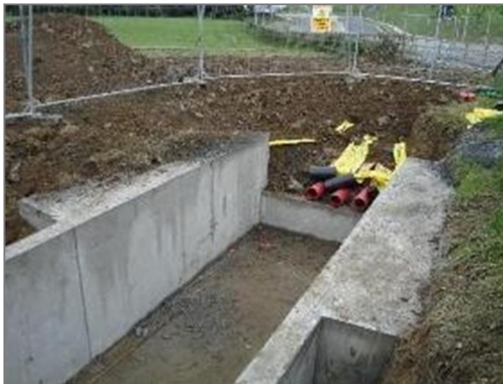
Figure 17 - Place pre-cast concrete sections on sand bedding.
