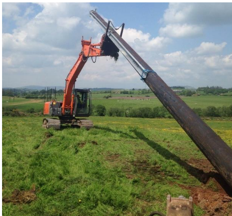
Figure 3 - Poleset removal with 13 Tonne excavator
