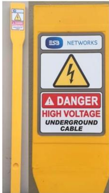
Figure 13 - Typical ESB Marker Posts
