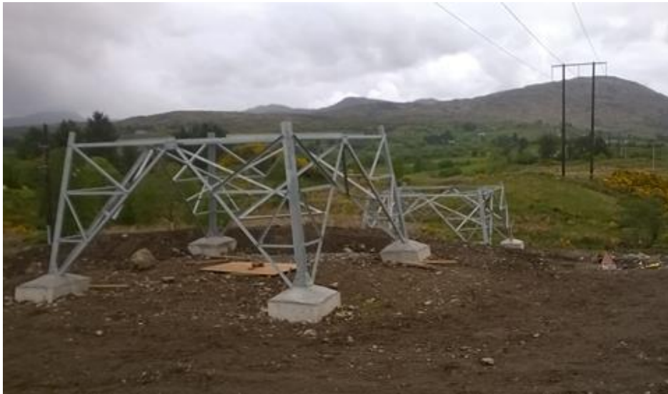
Figure 7 - 110kV Interface Mast foundation complete
