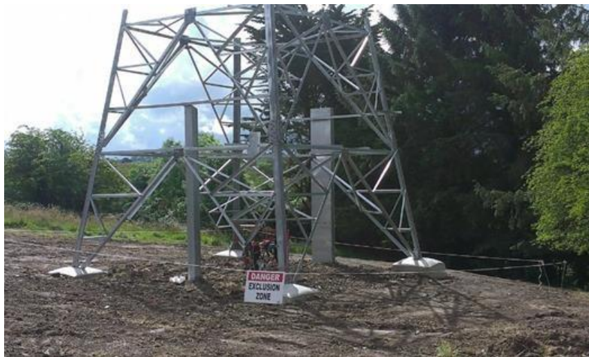
Figure 8 - Base of Interface Mast structure backfilled
